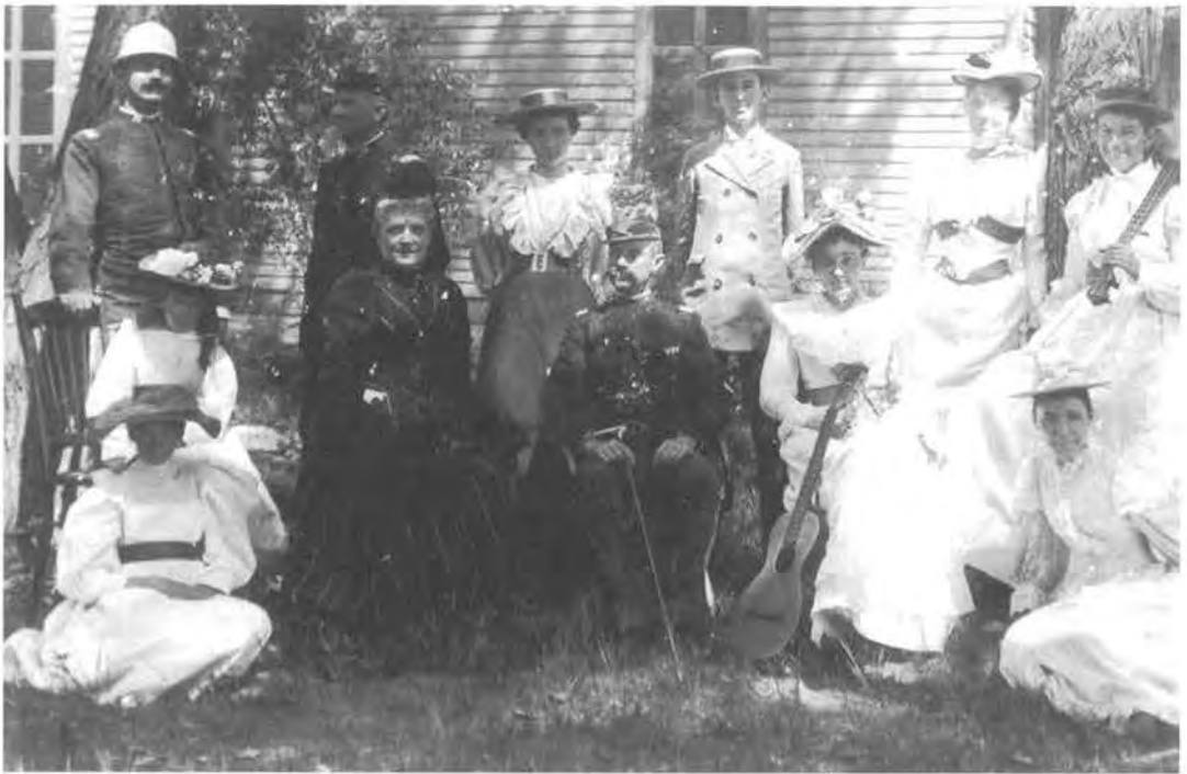
Residents of Fort Sidney, Nebraska, prepare for a concert on the lawn, c. 1890.
